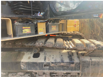
Image Comment(s): 2x missing track pads right side assembly
